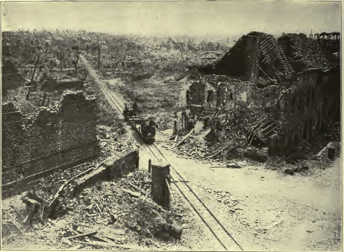
A tramway track, used to supply the Canadian Corps, running through the ruins of a French village destroyed by German shell-fire. Narrow-gauge roads like this, operated by motors, proved invaluable in bringing up supplies and moving the wounded to the rear. (Canadian official photograph.)
